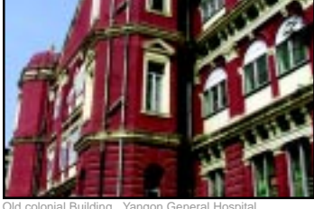
Old colonial Building , Yangon General Hospital
